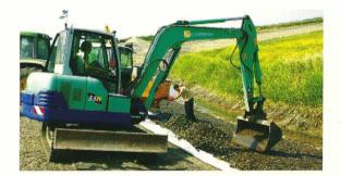
Elastocoast can be placed in-situ using local aggregate to minimize environmental disruption and reduce construction costs. Offering design flexibility, Elastocoast can be uniquely formed into a monolithic structure to best fit the environment.
